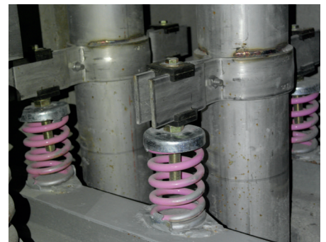
SPRING MOUNT INSTALL DETAIL
